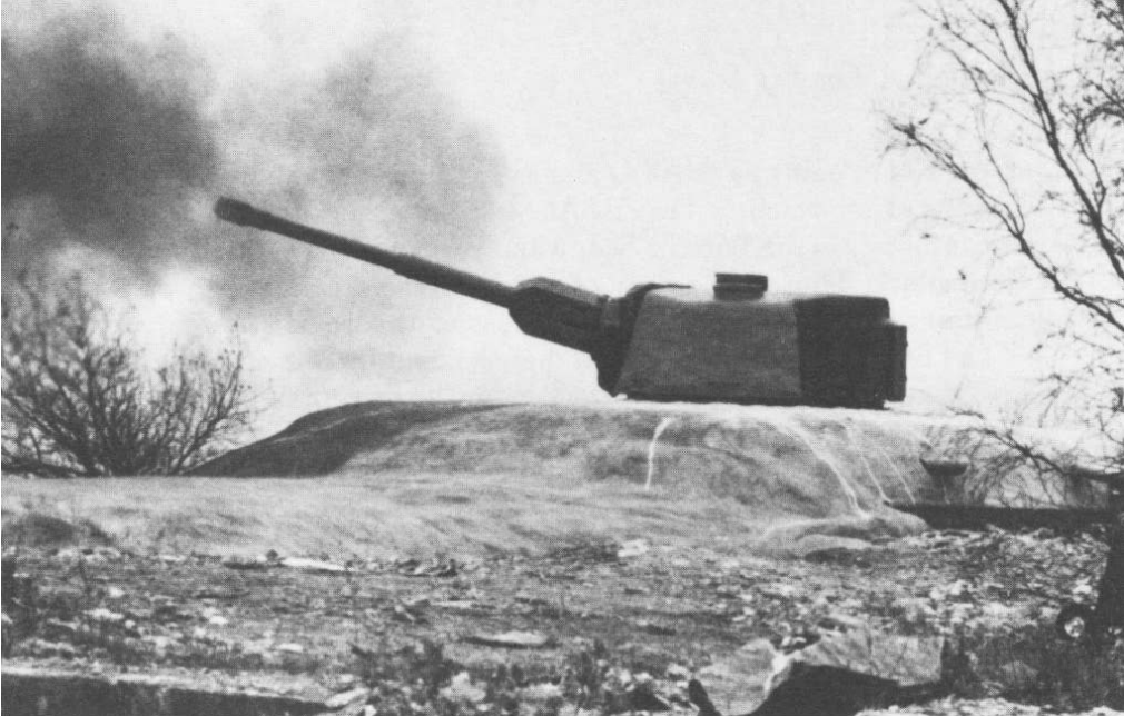
Finnish-made 130mm "turret cannon" firing in reinforced coastal artillery emplacement Courtesy General Headquarters, Finnish Defense Forces
