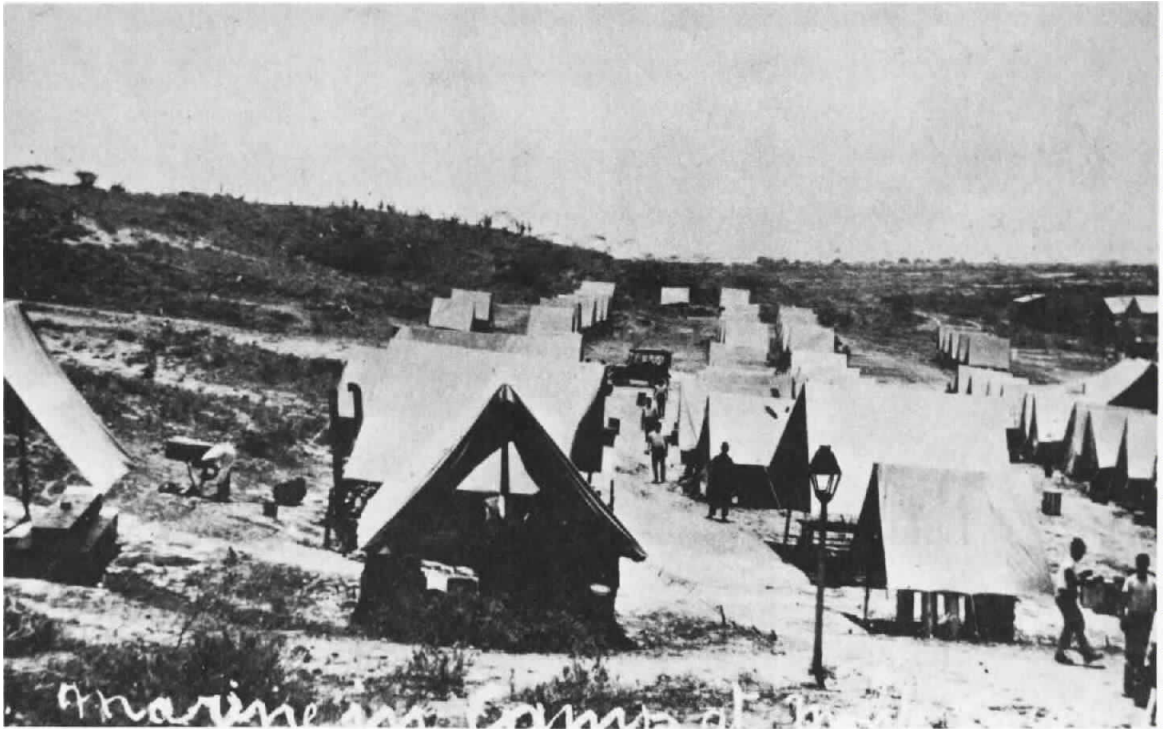
Marine camp at Monte Cristi, complete with street lamp and automobile.
