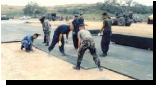
Marines Laying AM-2 for an EAF
