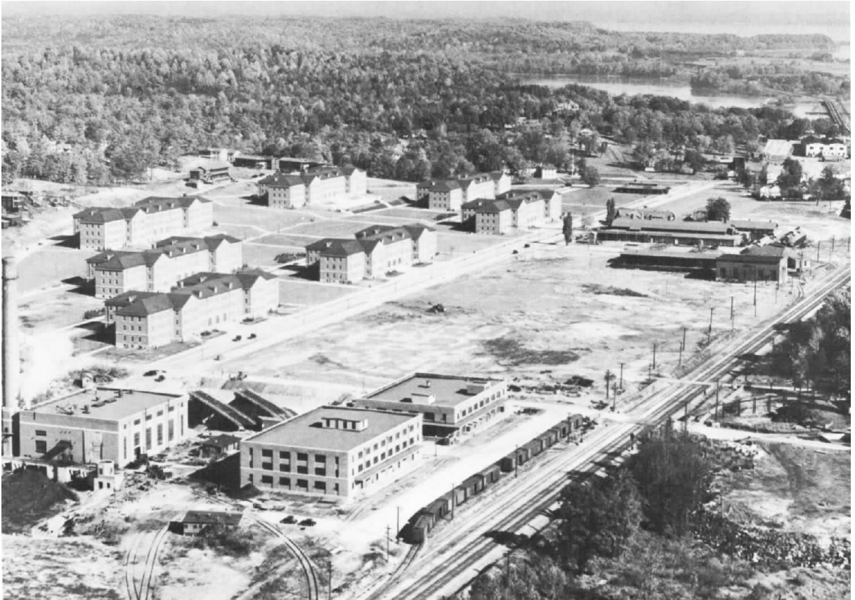
By November 1932, the new barracks were completed and Barnett Avenue (with the vehicles on it) had been relocated. (USMC Photo 529015).
