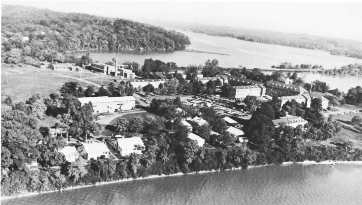
The Naval Hospital, Quantico (right center) and supporting buildings, located on Shipping Point. Quantico Creek is above the complex and the Potomac River below. (Quantico Photo 012-3523-54-76).
