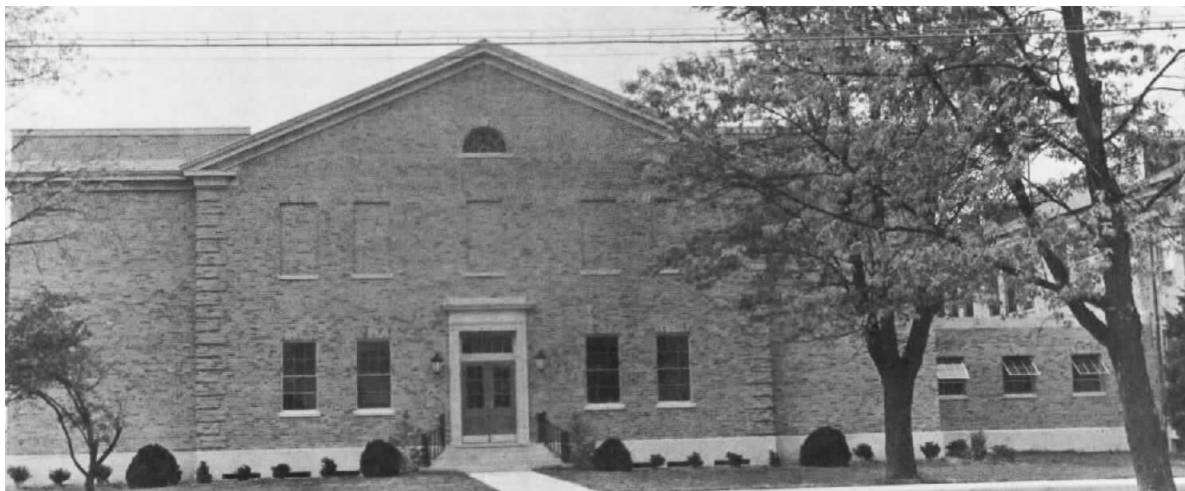
Ellis Hall, an important amphibious warfare training facility within the Education Center. (USMC Photo A308924).
