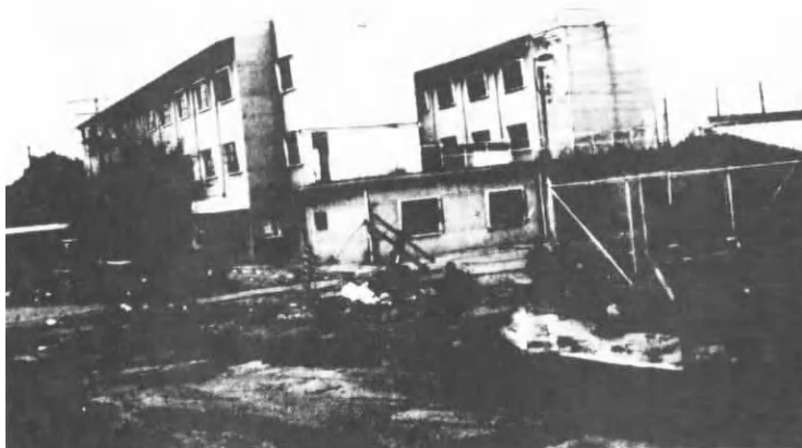
Landing zone in PX compound.
