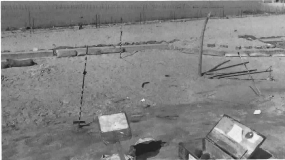
The Iraqi beach defenses looking seaward from a mortar emplacement. Striped rods are aiming stakes. There are three lines of barbed wire entanglements: one is in chest-deep water near top of picture and two more are at the edge of the water, with mines in between. In the middle is part of an interlocking trenchline network built with concrete blocks and highway K-rail. Adjacent bunkers contained antitank rockets and grenade launchers.
