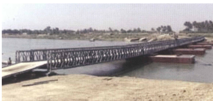
The MEG emplaced Maybey-Johnson bridges over water obstacles where a more permanent structure was required.
