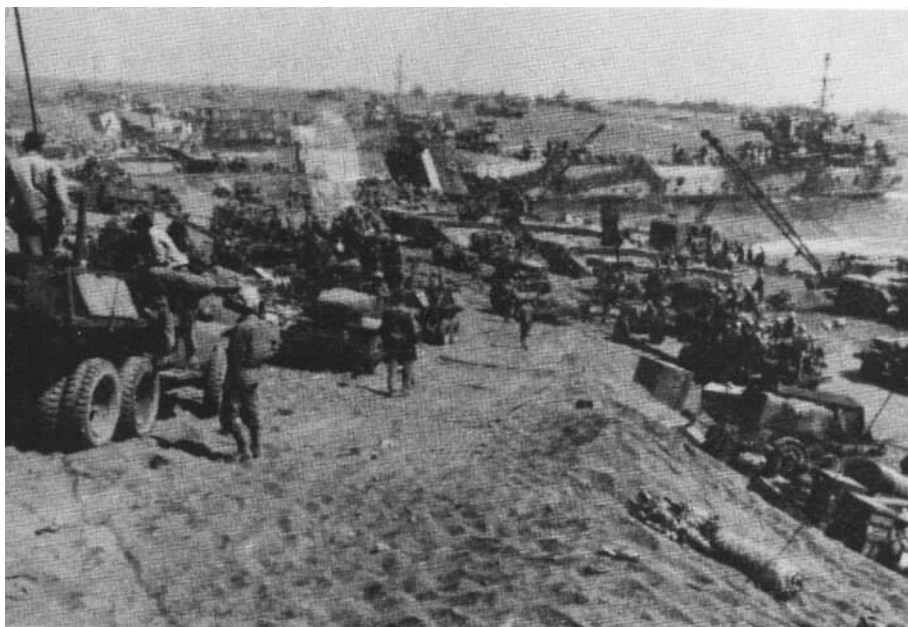
Preassembled Marston matting is laid.
