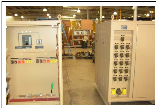
Figure E-9. Secondary distribution center
