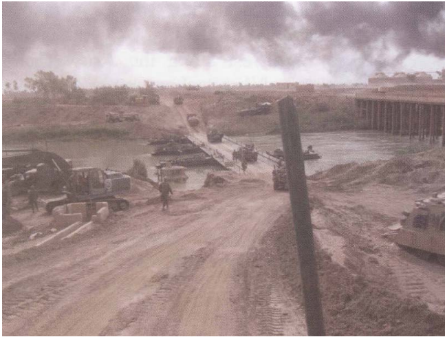
Engineers emplace a ribbon bridge over the Diyala River to speed the attack.
