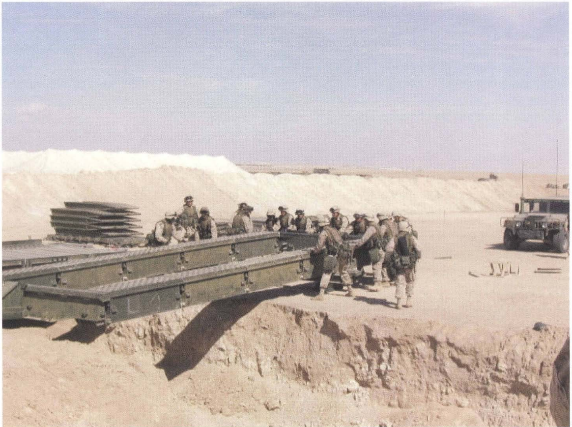
Marine Engineers created a full-scale mockup of the border obstacles to rehearse breaching and bridging techniques.
