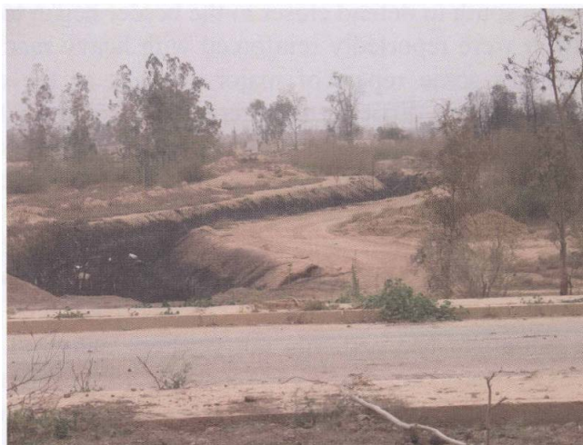
'Fire Trenches' were dug by the Iraqis. When filled with oil and set ablaze, they provided obscuration of defensive positions and artillery systems.
