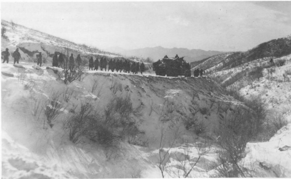
A unit of Company C, 7th Marines, led by senior regimental commander Col Homer L. Litzenberg, Jr., moves out to repair a downed bridge south of Koto-ri during the 1st Division's "attack in a different direction" of early December 1950.
