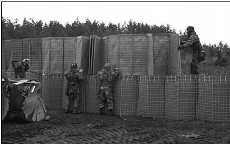
Figure 8-11. Wire and fabric container revetment
