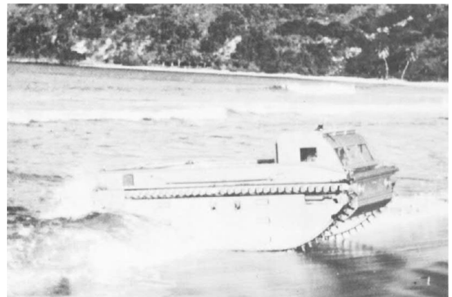
The "amphibian tractor" of the Navy Department's Bureau of Ships, the famous "fourth model" of the Alligator, was photographed undergoing tests in 1940 in the Caribbean Sea.
