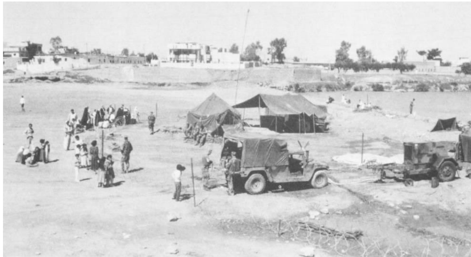
Marine engineers from MSSG 24 are busy constructing a water distribution point on the banks of the Khabur River in Central Zakho. Clearly visible are a portable electrical generator, the Reverse Osmosis Water Purification Units (ROWPU) holding tanks, and a field antenna. The compound is protected by a single strand of barbed wire. The Khabur River is a tributary of the famous Tigris River which runs from the Taurus Mountains through Iraq to the Persian Gulf.
