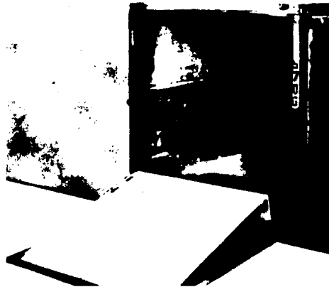
Figure 4-65. Mechanical ramp recessed in the loading dock.
