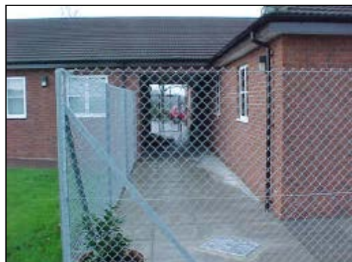
Figure K-5.--Facility Walkway
