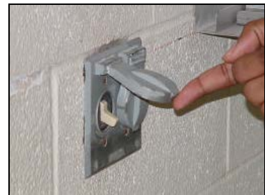
Figure K-16.-- Waterproof Fixture
