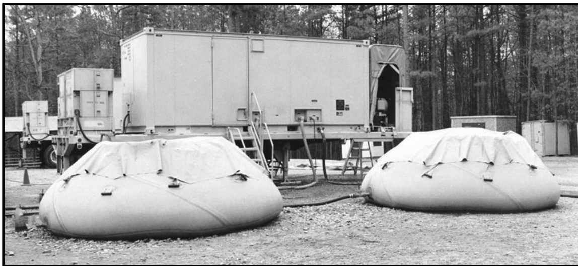
Figure A-3. Reverse osmosis water purification unit
