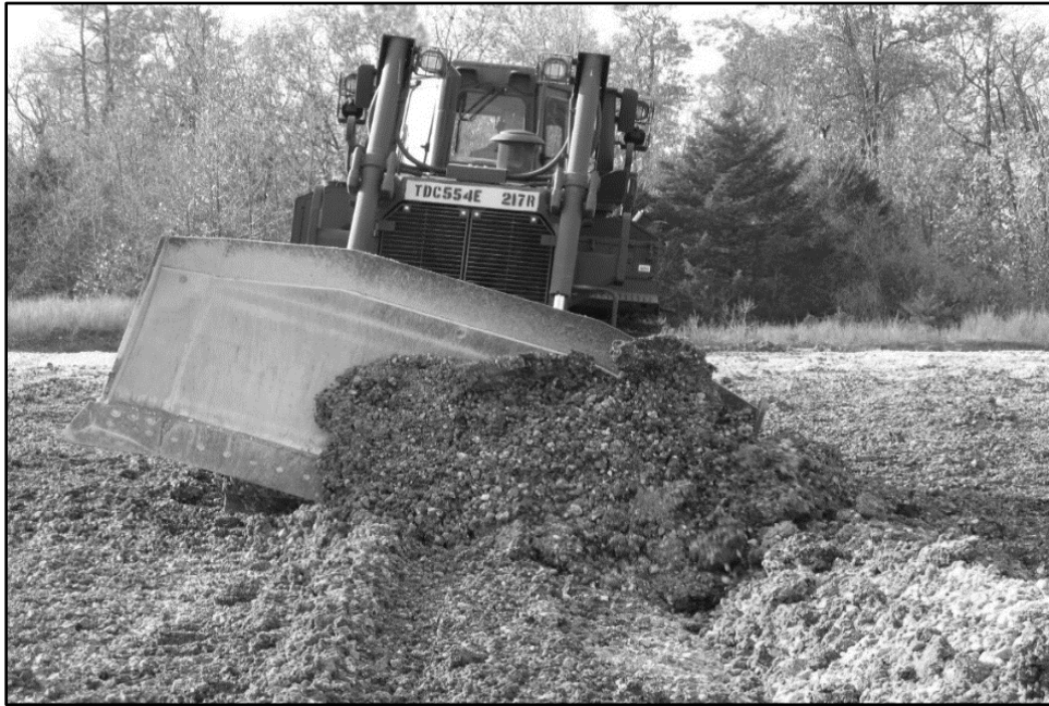
Figure 2-11. Tilt dozer ditching
