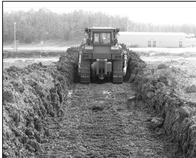
Figure 2-9. Slot dozing
