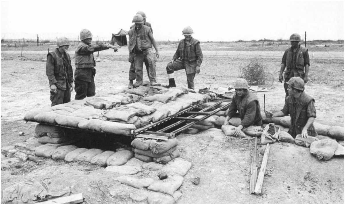
Top is Department of Defense (USMC) Photo A190200 and bottom is Department of Defense (USMC) Photo A190197. Marine engineers with a bulldozer are building ammunition storage bunkers at Combat Base Area C-4, top, and a Marine platoon from the 1st Battalion, 4th Marines is seen at work building a bunker emplacement at C-4 with sandbags for overhead cover in January, bottom.
