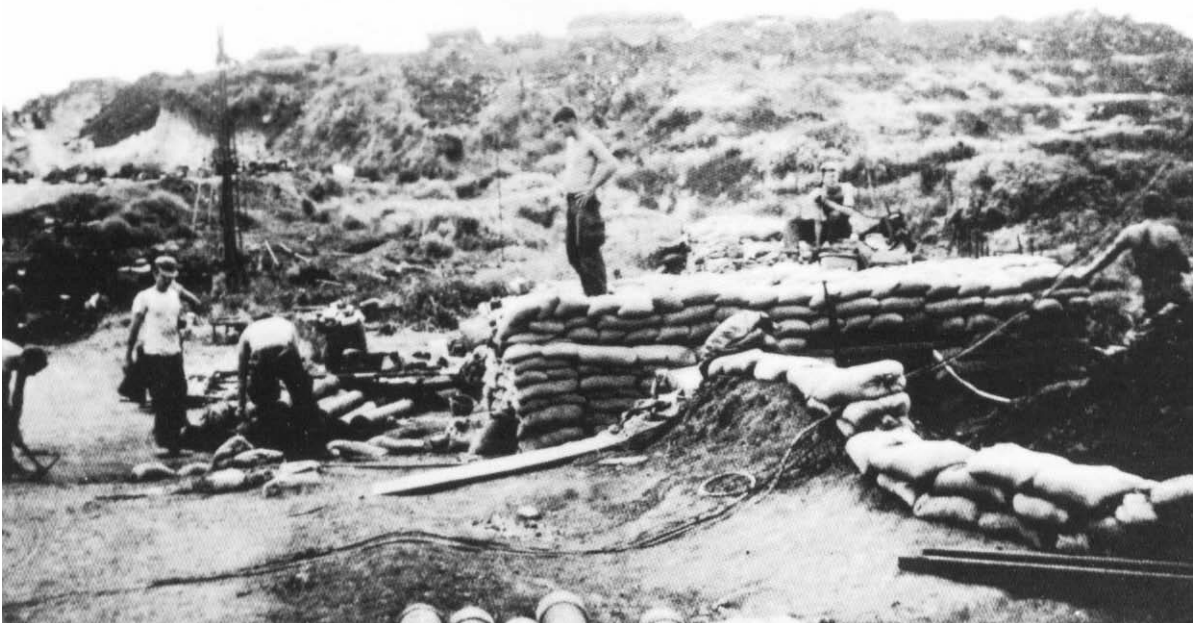
Top photo courtesy of Col Joseph L. Sadowski, USMC (Ret), and bottom photo courtesy of Col Lee R. Bendell, USMC (Ret) The Marine base at Con Thien (A-4) is seen at top, with Marines constructing bunkers at A-4 in photograph at bottom. Col Lee R. Bendell, whose 3d Battalion, 4th Marines served at Con Thien in 1967, observed that NVA artillery fire "necessitated overhead protection."
