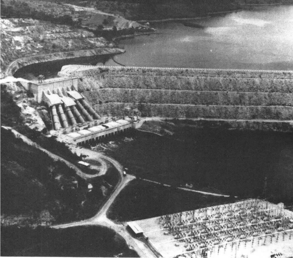
Hydroelectric sluices in the Akosombo Dam Courtesy Embassy of Ghana, Washington
