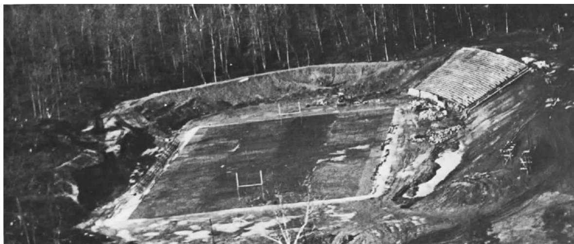
Butler Stadium, a self-help project of the first order, was literally carved out of forest, rock, and earth by Butler's Marines. (Don C. Micheau Collection. Personal Papers Section, Marine Corps Historical Center).
