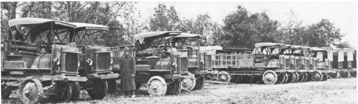
Jeffery Quad cargo trucks at Quantico in 1918. During the fall rains, the unpaved streets became a quagmire of mud that required the use of chains on the solid rubber-tired wheels. (USMC Photo 518095).
