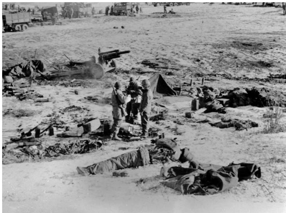
Photo courtesy of Sgt Norman L. Strickbine, USA East of the reservoir during 28 November, the Army's 3d Battalion, 31st Infantry, and two firing batteries of the 57th Field Artillery Battalion painfully reorganized after the previous night's devastating attack against their positions just south of Pungnyuri Inlet. Bodies can be seen in the foreground. Sporadic fighting continued north of the inlet.
