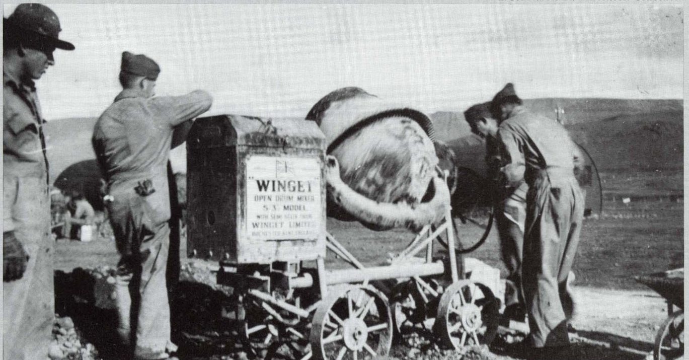
Marines constructing Nissen huts mix cement in an old mixer for their foundations.
