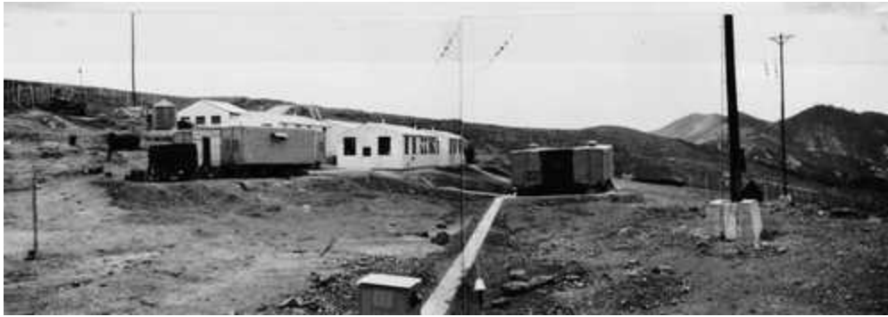
Coast Guard LORAN Station Pusan, code-named Elmo #4 near Pusan, South Korea in November, 1952. The Coast Guard quickly built the base and put it into operation to satisfy the need for adequate navigational services to United Nation's forces during the conflict.
