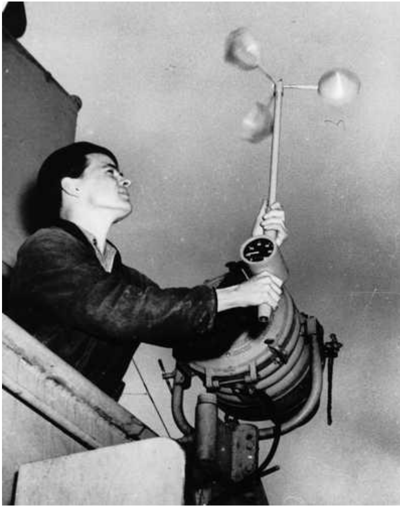
A crewman determines the velocity of surface winds by the use of an anemometer, one of the many instruments utilized by the ocean station cutters.
