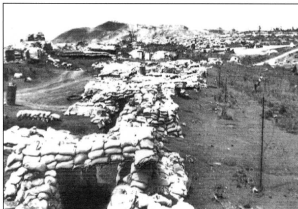
Bunkers along the trench line that ringed the combat base. The innermost defensive wire barriers can be seen on the right.
